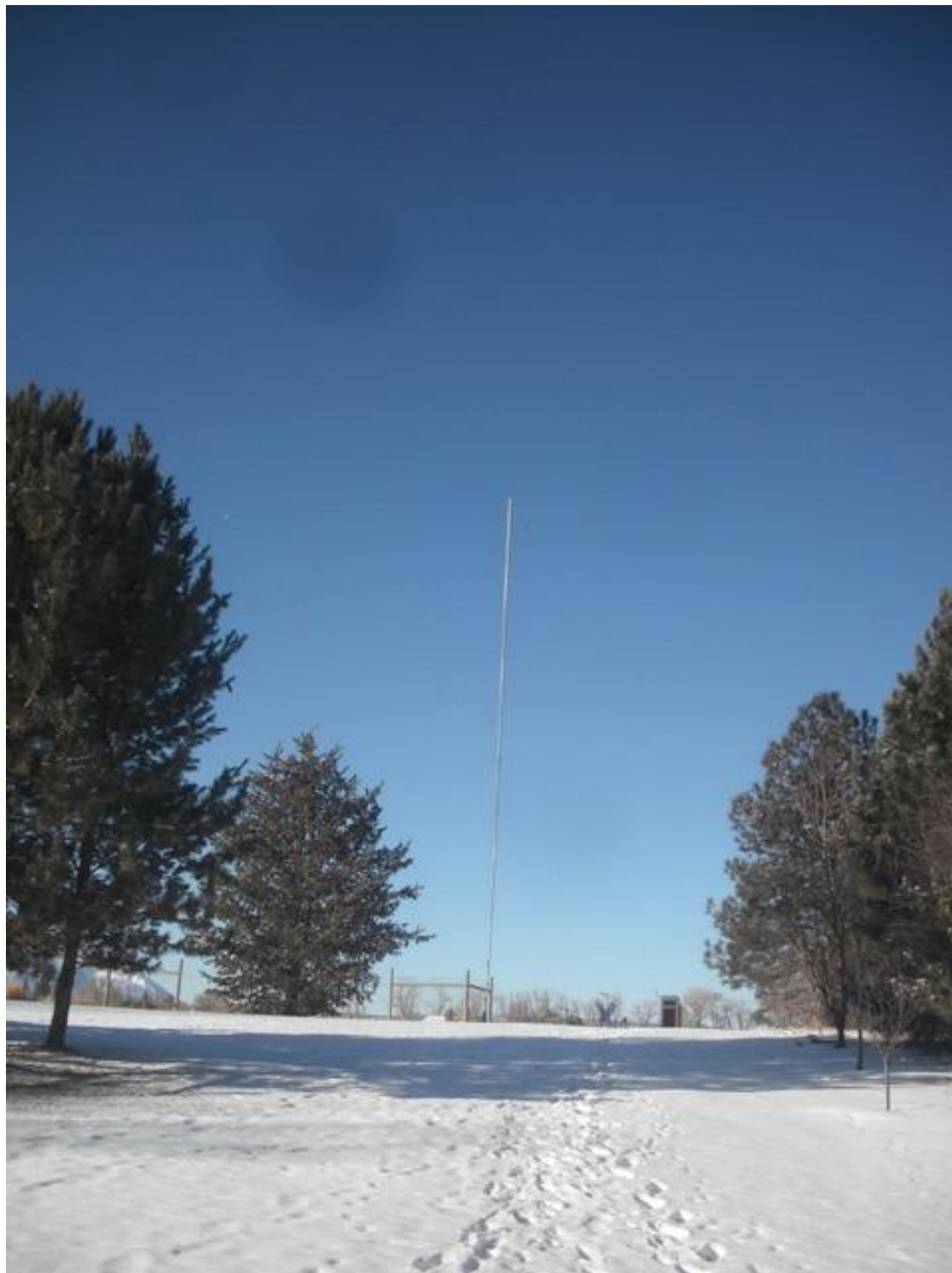
Antenna and Helix Hut
