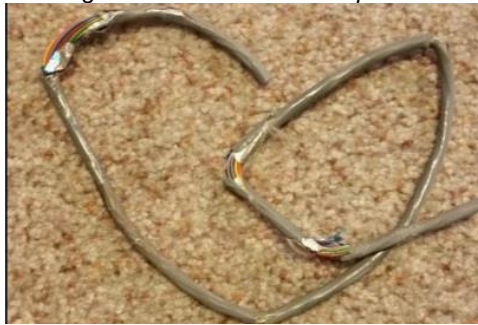
Damaged Control Cable from top of Tower
